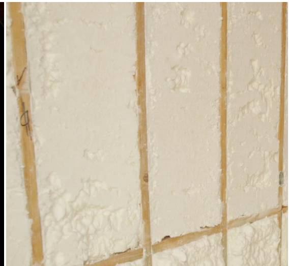
Figure 4: Typical appearance of shaved SPF (be aware that shadows in photographs can make uniform foam appear multiple colors in photographs).
