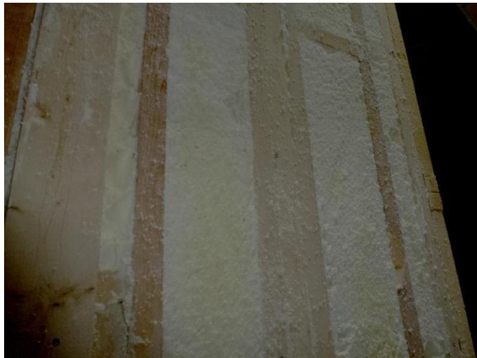
Figure 4: Typical appearance of shaved SPF (be aware that shadows in photographs can make uniform foam appear multiple colors in photographs).
