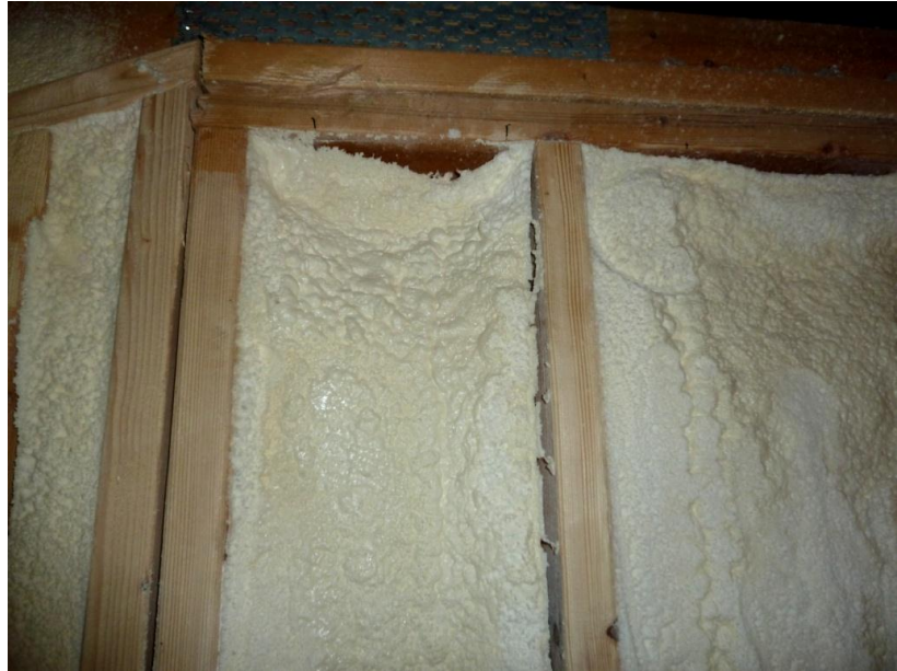
Figure 5: Foam shrinkage.
