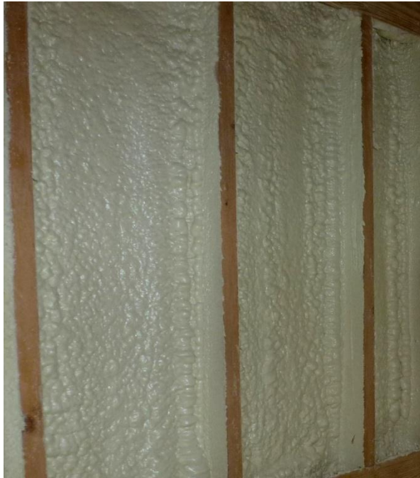
Figure 2: Typical appearance of closed-cell SPF.
