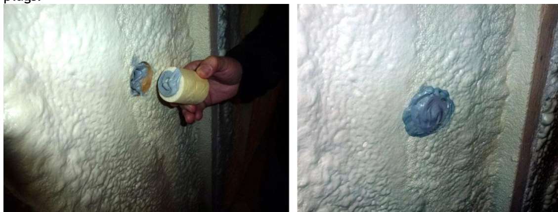
Figure 22: Repairing a core hole with plug and sealant.
