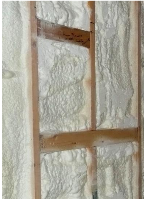
Figure 3: Typical appearance of open-cell SPF.
