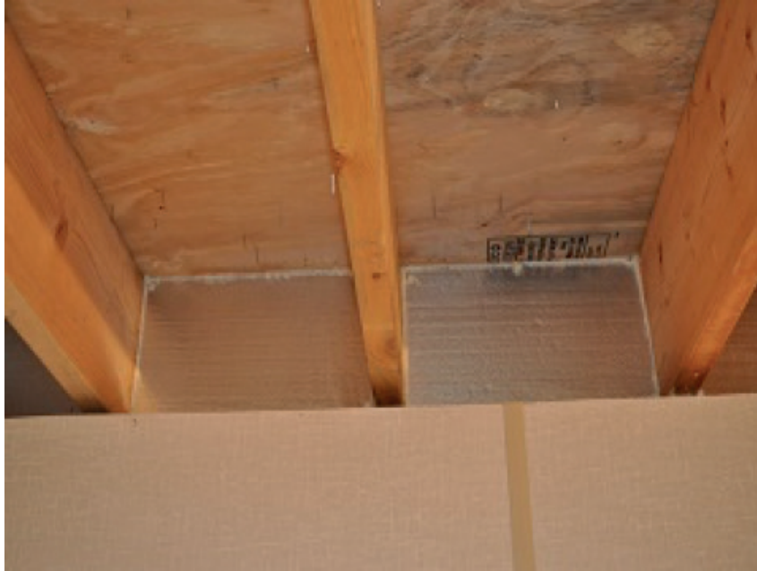
FIGURE 13. Foam board insulation and sealant/caulk at the foundation-framing area
