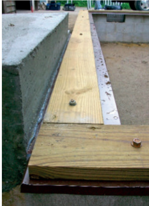
FIGURE 10. Physical termite barriers and shields
