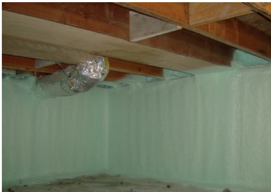
FIGURE 15. SPF insulation of a conditioned crawlspace wall
