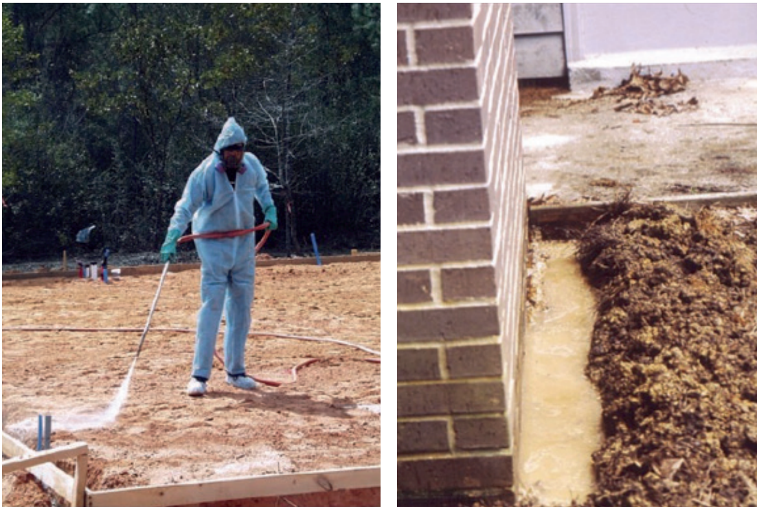
FIGURE 7. Termiticide treatment of the ground below slab and near the foundation
