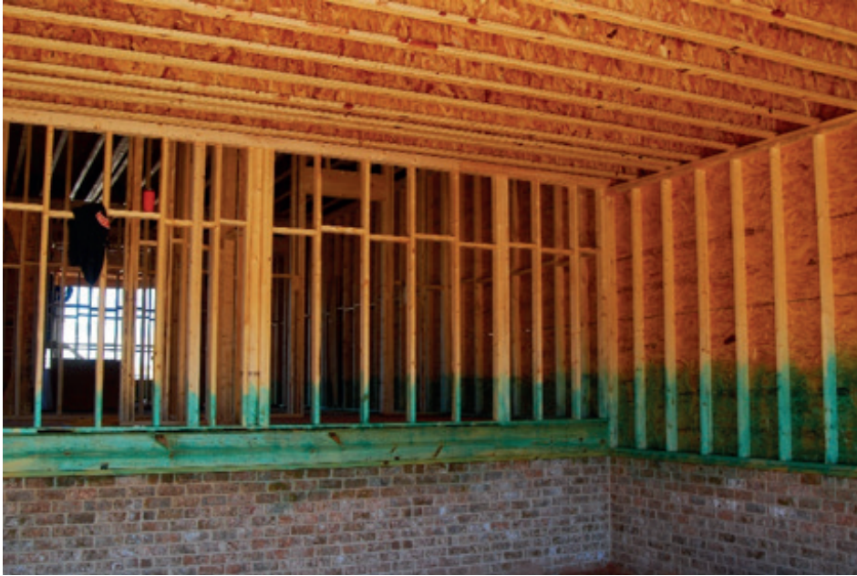
FIGURE 6. Borate treatment of select structural wood components
