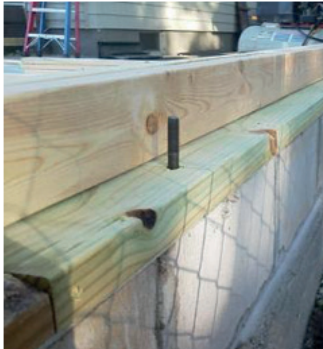
Courtesy of Root River Inspections
