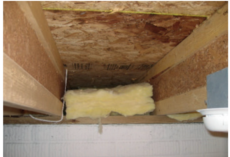
FIGURE 14. Sealing and insulating the band joist with fiberglass batts (improperly re-installed)
