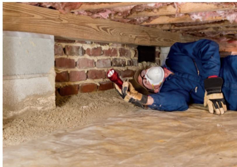
FIGURE 3. Visual termite inspection
