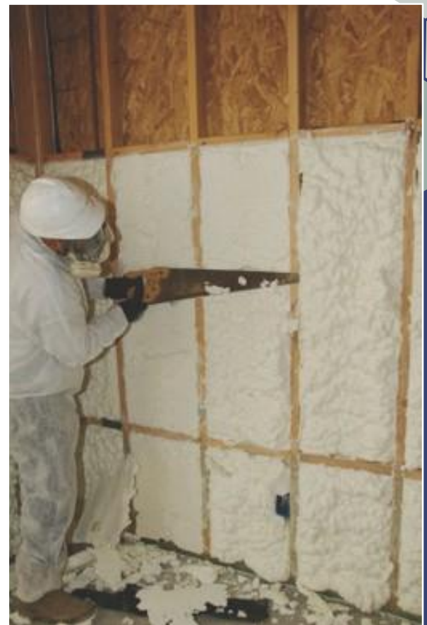
Figure 15: Contractor trimming foam
