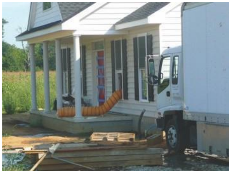
Figure 12: Provide adequate ventilation
