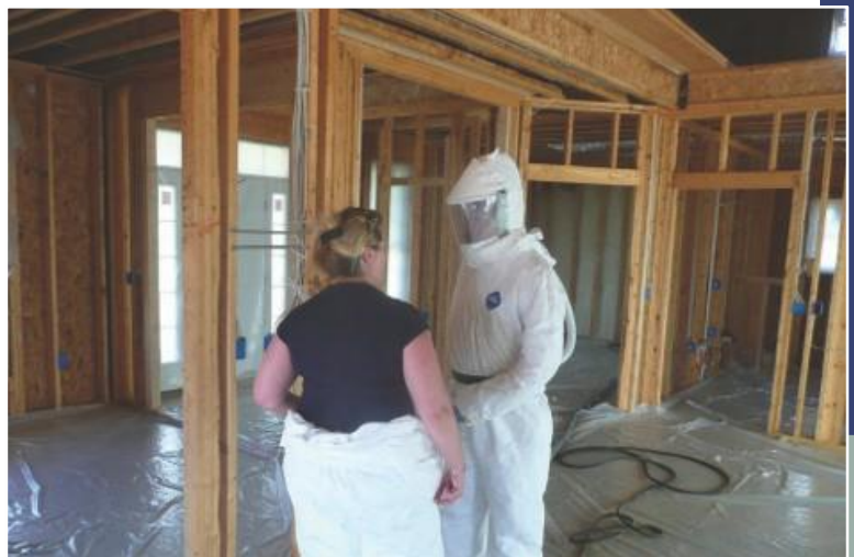
Figure 11: Provide notice to trades and occupants
