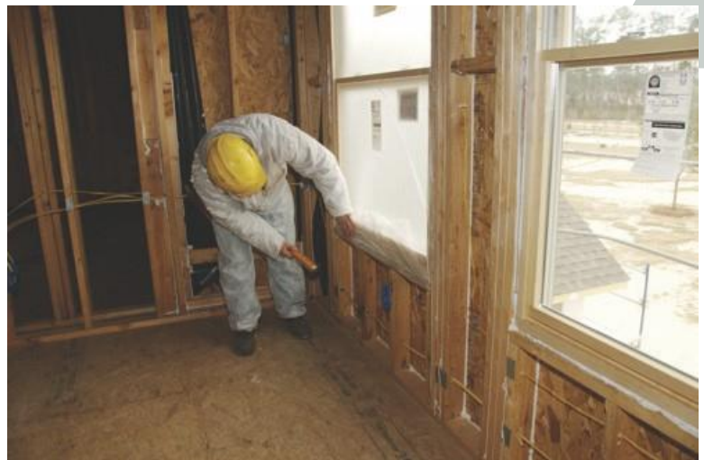
Figure 10: Sealing the windows
